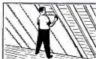
Shows how to apply rugged Gold Bond Rock Wool Blankets between rafters of floored attic.
